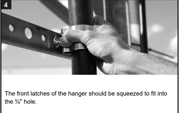
The front latches of the hanger should be squeezed to fit into the 3/4" hole.
