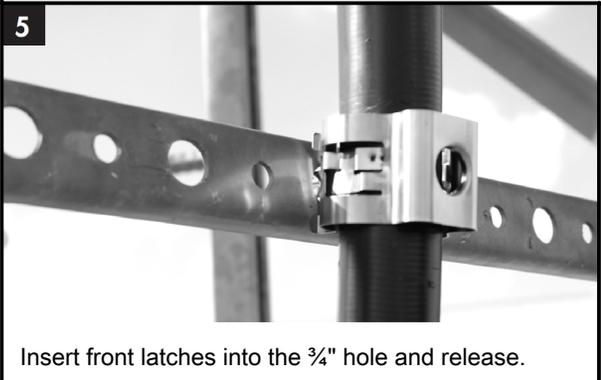
Insert front latches into the 3/4" hole and release.
