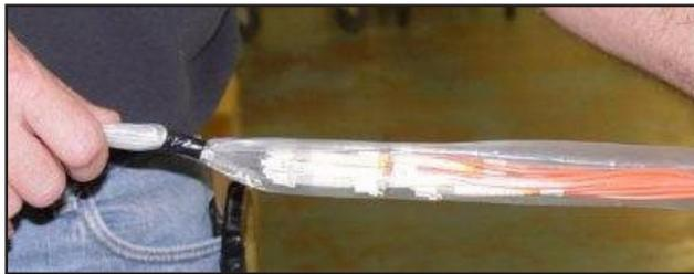
After you have pulled the fiber and power conductors into the OVP box remove electrical tape from the trunk cable and remove clear tube for access to all optical connectors.
