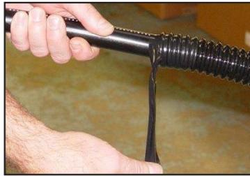
Remove electrical tape from the trunk cable and corrugated protection tube
