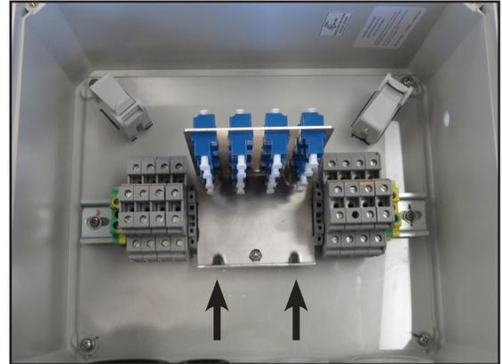
2. Install Multimode hybrid trunk cable in the black gland, bottom left corner. Tighten the external gland nut to hold the cable in place.
