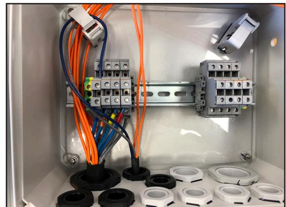
4. Install Multimode or Single mode hybrid jumper cable in the small black gland, center. Tighten the external gland nut to hold the cable in place.
