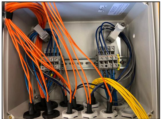
14. Install Single mode hybrid jumper cable in the small white gland, top fourth from the left. Tighten the external gland nut to hold the cable in place.
