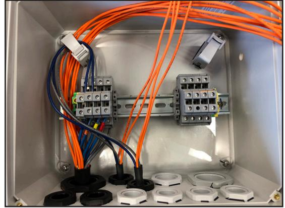
5. Install Multimode or Single mode hybrid jumper cable in the small black gland, top left. Tighten the external gland nut to hold the cable in place.
