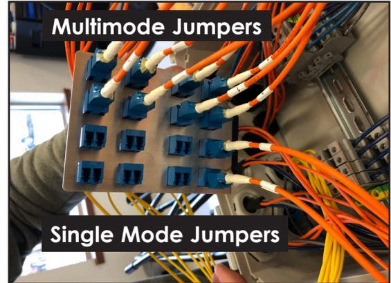
17. Carefully slide fiber patch panel back into its original slot being sure that no furcation tube are trapped between the rail and power terminals.
