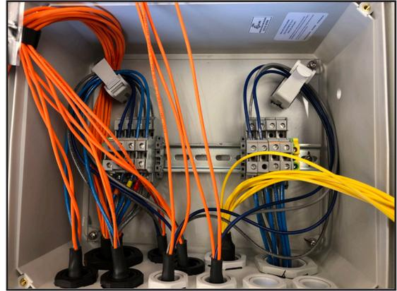
13. Install Single mode hybrid jumper cable in the small white gland, top third from the left. Tighten the external gland nut to hold the cable in place.
