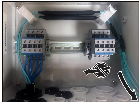
3. Install Multimode or Single mode hybrid jumper cable in the small black gland, bottom left. Tighten the external gland nut to hold the cable in place.
