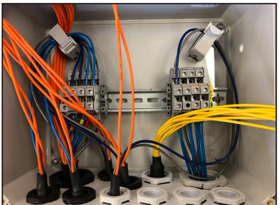
12. Install Single mode hybrid jumper cable in the small white gland, top second from the left. Tighten the external gland nut to hold the cable in place.
