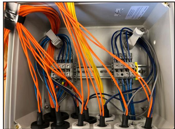
15. Picture A: Connect the Single Mode trunk DLC fiber connectors to the fiber patch panel as shown. Starting from the bottom outside left with #1 and #2 next to it. Next row up will have #3 outside left and #4 next to it. Continue until fully populated.
