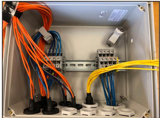
11. Install Single Mode hybrid jumper cable in the small white gland, top left. Tighten the external gland nut to hold the cable in place.
