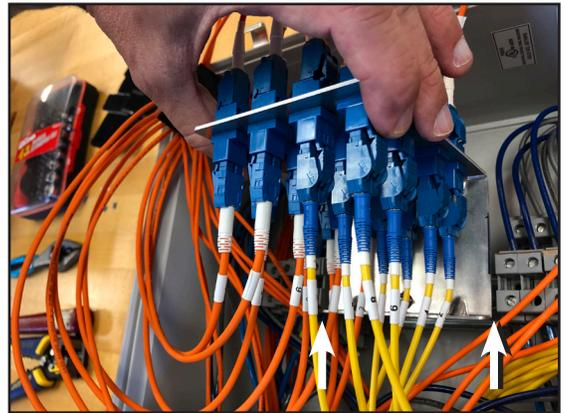
18. Hook the bottom of the bracket on the rail, push forward while tipping the patch panel away from yourself, lower the patch panel to engage the front locking clips.
