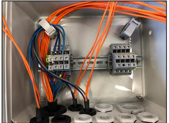
6. Install Multimode or Single mode hybrid jumper cable in the small black gland, top second from left. Tighten the external gland nut to hold the cable in place.
