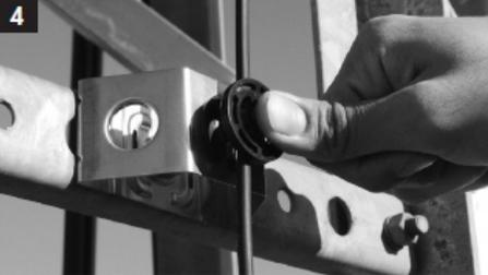
Push SnapStak hanger in tower member or mounting adapter with 3/4" hole.
