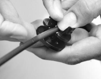
Push cable into the support channel with finger or thumb while expanding hanger latches.
