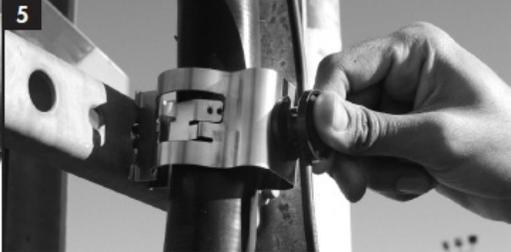
Plastic SnapStak hangers may be snapped into any other CommScope metal or plastic SnapStak hanger size.
